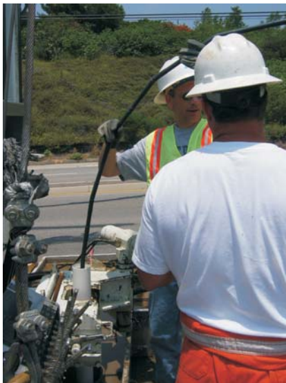
Figure 3. Installation of the SAA for unstable slope monitoring in California
