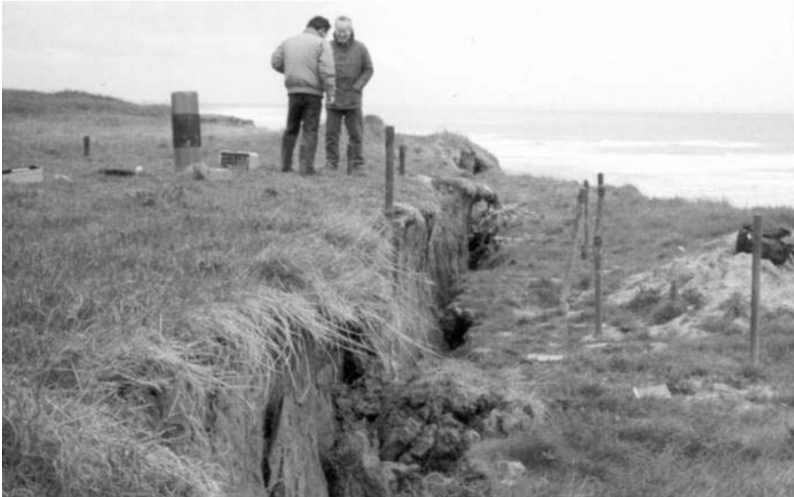
Figure 1. View of slope failure at Cowden, located through centre of instrument array (Dixon et al. 2003)
